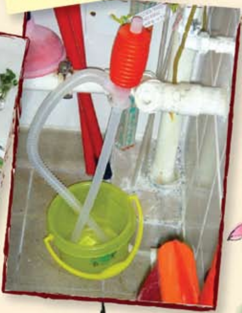
Workers made use of pumps and pipes to avoid direct contact with organic solvents and reduce exposure to chemical vapours.
